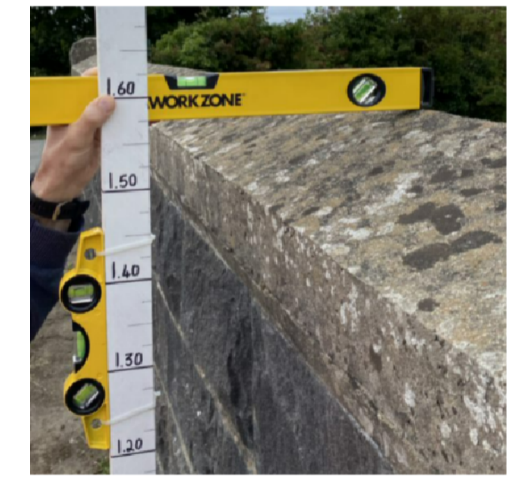
OBB41 PARAPET IMAGE 000740
